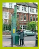
Q3: Stink Pipe. These pipes provided ventilation for the sewage system built in Victorian times. They prevented the build up of gases. Why do you think it is built to be higher than people?
